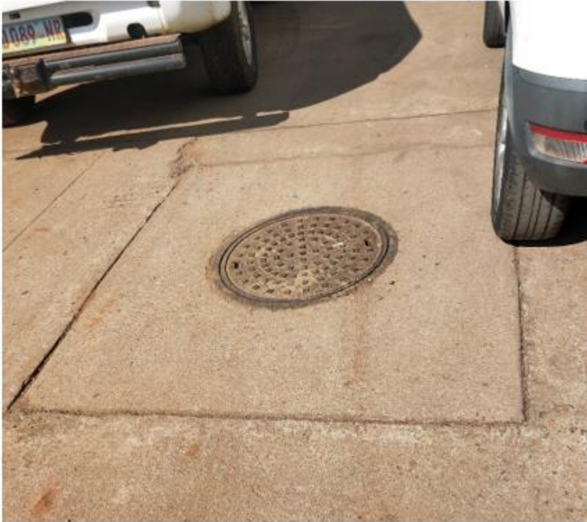
Photo plate 1: Manholes at the proposed site
